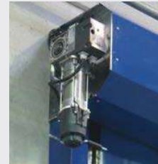
Gear motor attached to door's frame
