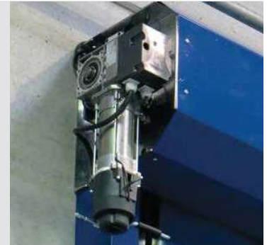
Gear motor attached to the frame
